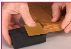
11. After curing, sand the damaged area.
