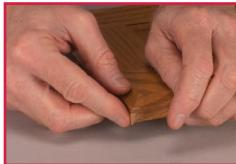
7. Force the epoxy material into the damaged area.
